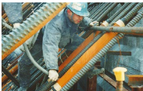
(Upper left) NMB Splice Sleeves for D51 bars
