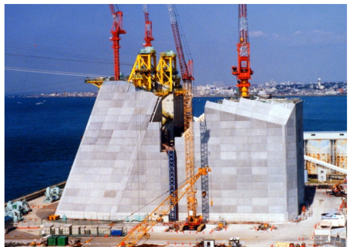
Anchorage 1A under construction
