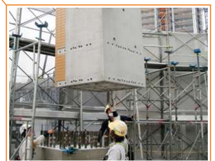
Precast column erection
