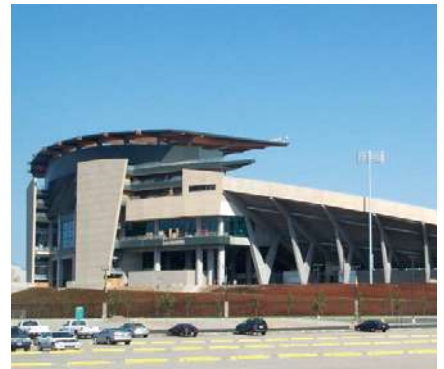
Autzen Stadium, U.S.A.
