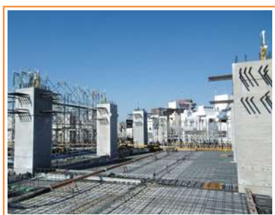
Precast column installation
