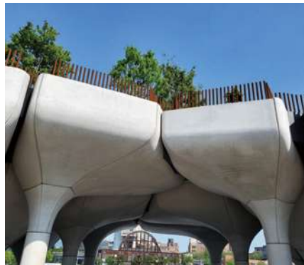
Little Island Pier55, U.S.A.
