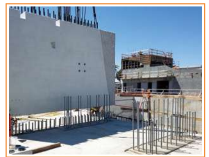
Precast wall installation
