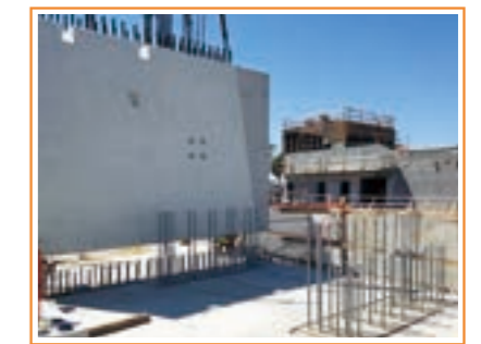
Precast wall installation
