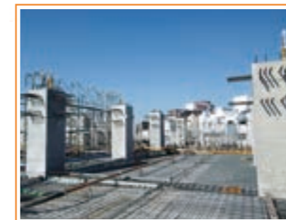
Precast column installation
