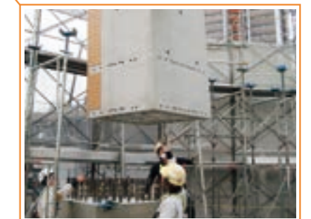
Precast column erection
