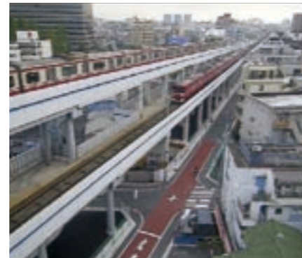
Elevated Railway, Japan
